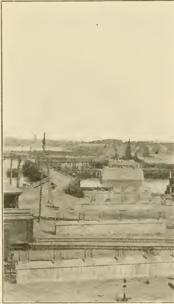
FIG. 7. VIEW FROM BRACKETT STEEET SHOWING PIERS AND TEMPORARY BRIDGE.
